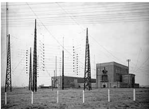
VLF aerial feed for Radio Station GBR Located at Rugby in England
