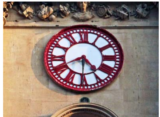
A clock with two minute hands, to show both GMT and local solar time.
