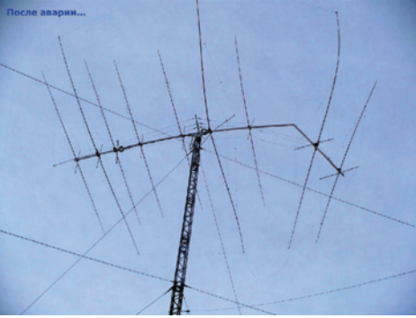
13. Showing the damage caused by ice and wind...
