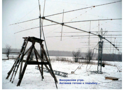
20. Sunday morning. The antenna is ready to erect.
