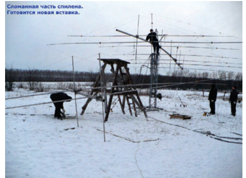
16. The broken part of the antenna is sawn off. The new insert prepared...
