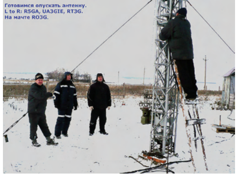
14. All are helping to lower the antenna a 3 el. Full size beam for 40m. metres and and so on...)
